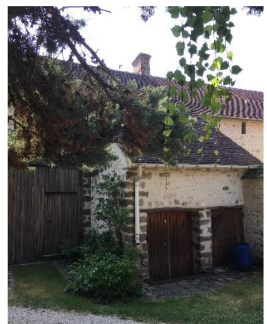
Figure 37 Exemple de descente de cave, 2018, © EG
