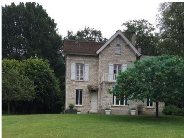
Figure 38 Villa rue de Larchant, 2018, © EG.
